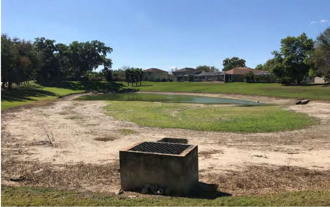
Photo 5 Southernly View of Pond 10
