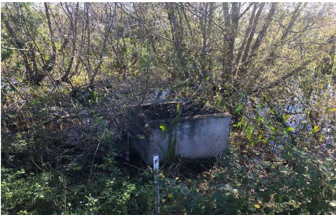
Photo 18 View of OCS 1500
