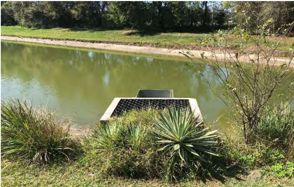
Photo 8 View of OCS 200
