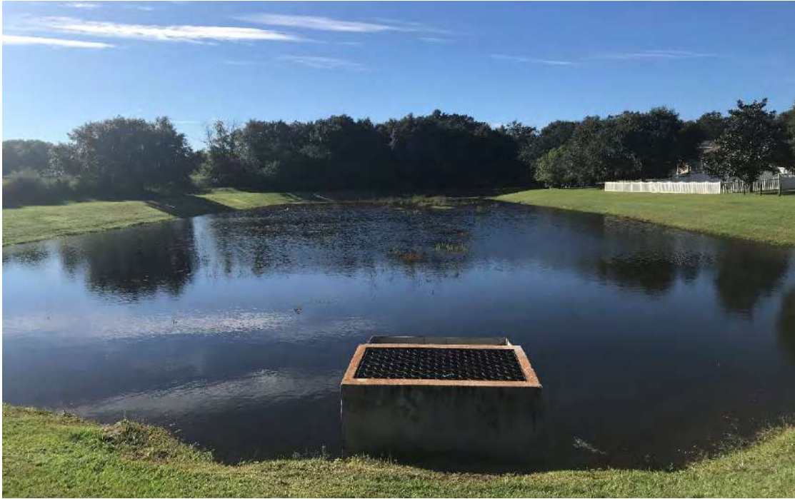
Photo 1 Southernly View of Pond 1000
