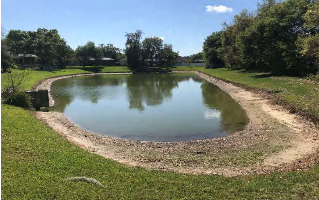
Photo 7 Southerly View of Pond 20
