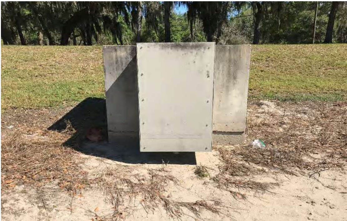
Photo 6 View of OCS 100 (Blocked Orifice)
