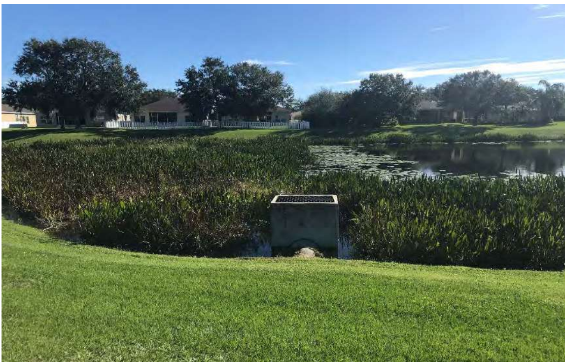
Photo 6 View of OCS 1200
