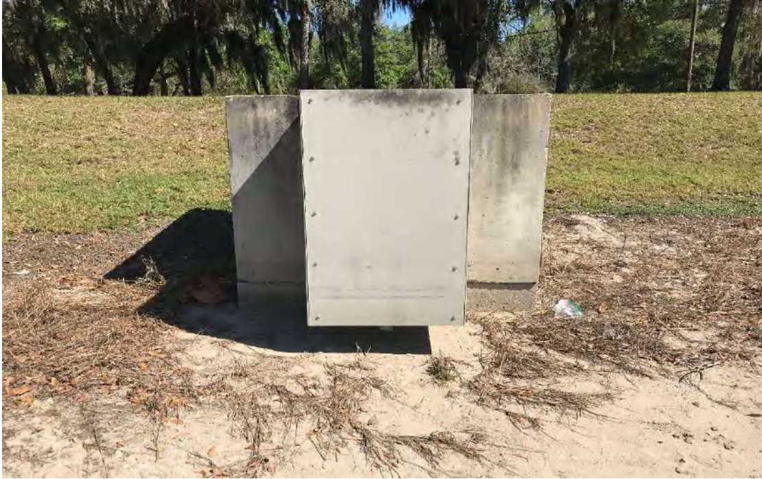
Photo 11 View of OCS 300
