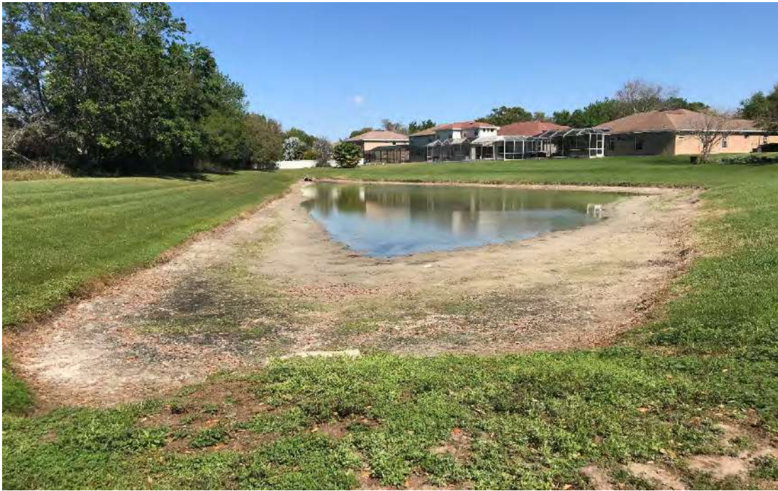
Photo 9 Northerly View of North Half of Pond 30
